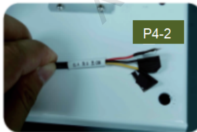
4. Modify the solar charge controller
